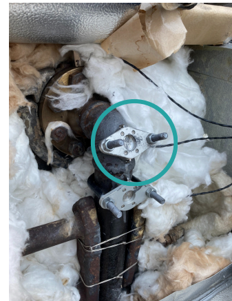
Figure 2. mPACT2WO's ultrasonic sensor on 2-inch elbow pipe
